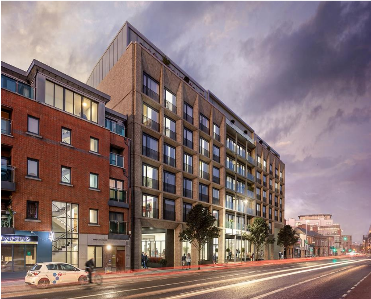
Development Ireland – Cork Street (Dublin) – 1.062 acre site located in Dublin City Centre -300 unit shared accommodation
