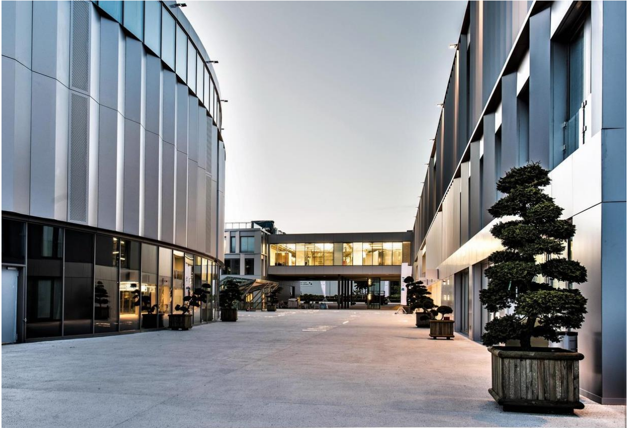
Commercial Income - iLife , in Etoy, is indicative of the Swiss Realtech investment strategy; this is a newly constructed complex of flexible office, education, restaurant and entertainment spaces. On acquisition, the team created a tailored asset management plan specifically addressing the tenant mix.
